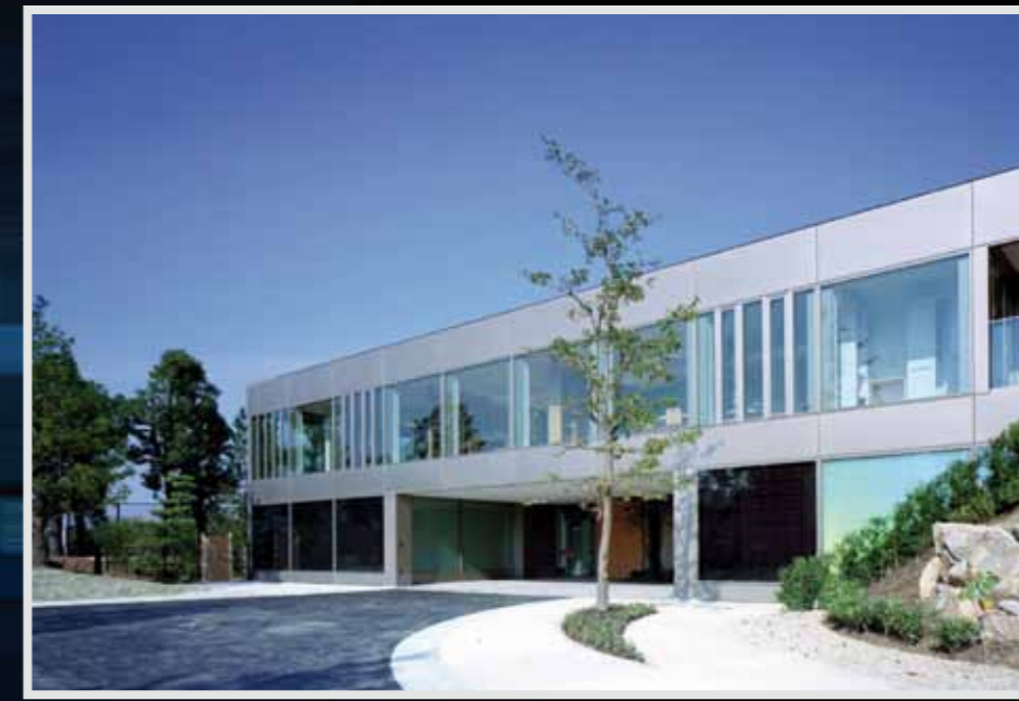
Figure-3 PAPI's exterior consists of aluminium frames and glass panels.
